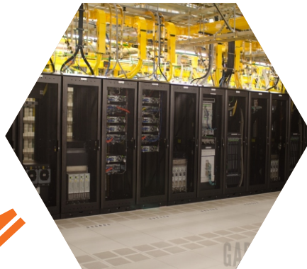
Fig. 1.2.8 Mobile Switching Centre
