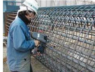
Fig 1.3.2: Bar bending work
