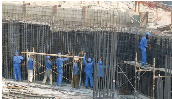
Fig 1.3.1: Bar bending and steel fixing work
