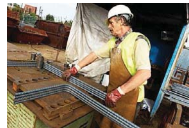
Fig 1.3.3: Bar bending work
