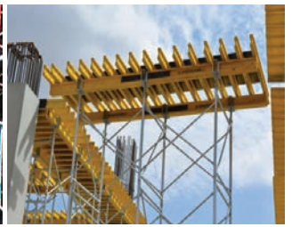
Fig. 1.2.14 System formed work
