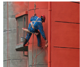
Fig. 1.2.16 Painting work by a painter
