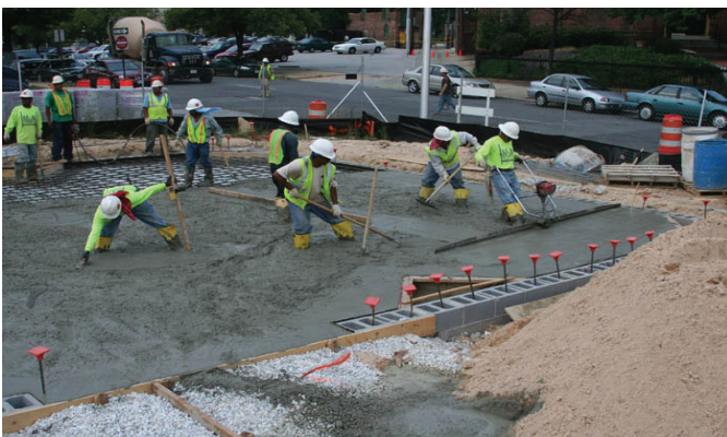
Fig. 1.2.9 Placing concrete
