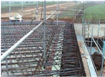
Fig. 1.2.11 Reinforcement bars fixed at site
