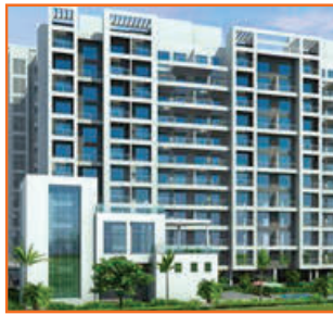
Fig:1.1.6: Residential Towers
