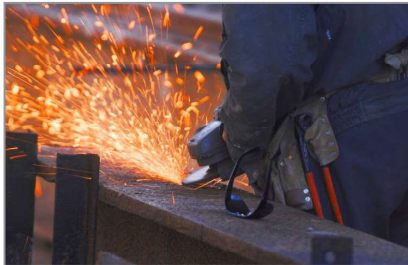
Fig. 2.1.5. LPG use at construction site
