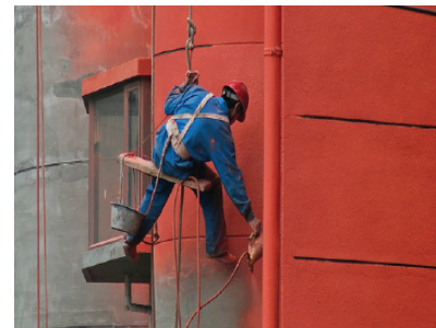
Fig. 1.2.16 Painting work by a painter
