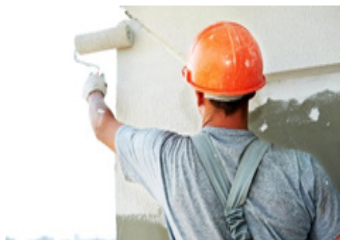
1.2.16. Paint work by a painter
