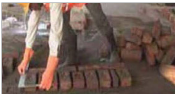
Fig. 1.2.1. Laying of bricks
