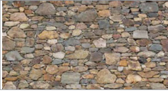
Fig. 1.2.3. Construct random rubble masonry
