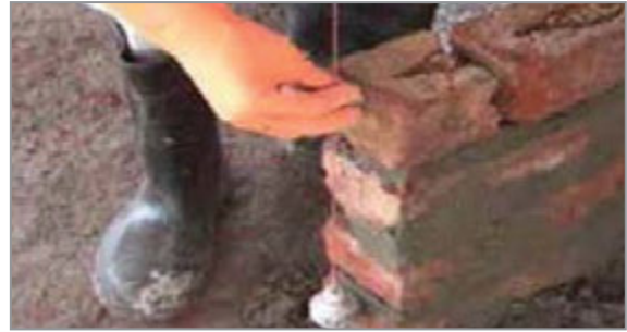
Fig. 1.2.6. Check alignment
