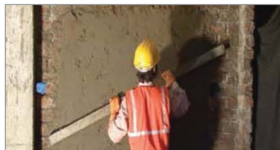
Fig. 1.2.2. Plastering
