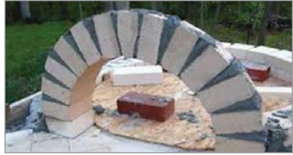
Fig. 1.2.4. Construct arches
