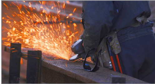
Fig. 2.1.5. LPG use at construction site
